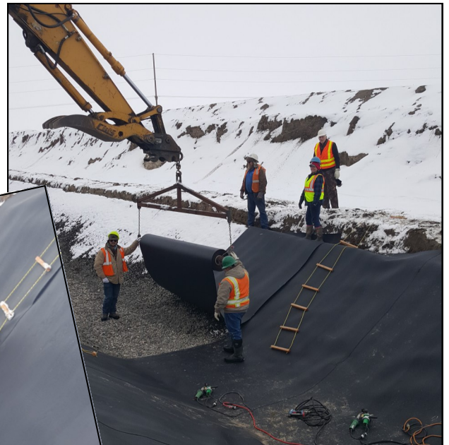
WEID Crew on March 1—Laying, stapling & hot welding the liner in place.
