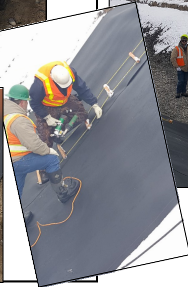
WEID Crew on March 1—Laying, stapling & hot welding the liner in place.
