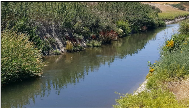
Coyote Springs seepage area Fall, 2019. Note green overgrowth and lack of canal structure. This is a high seepage area, due to springs impacting the canal.
